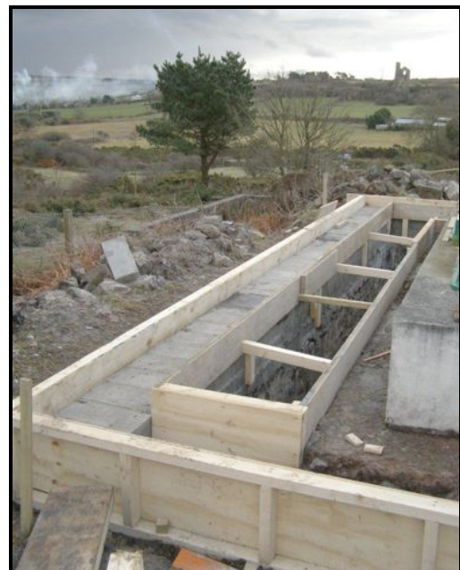
New foundation blockwork and shuttering February 2010
