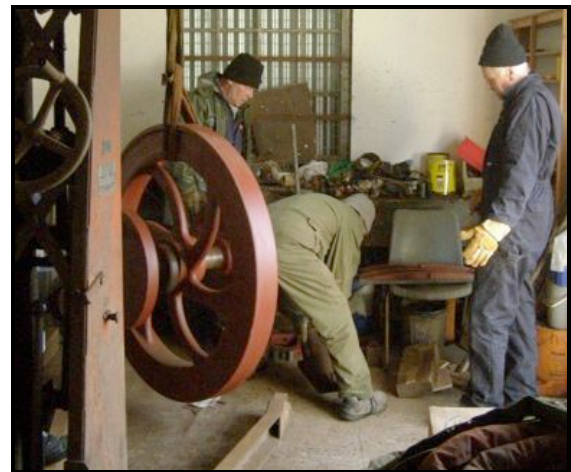
Cleaned and painted flywheel on hydraulic lift, Frank Kneebone, Huw Rowe and David Blight
