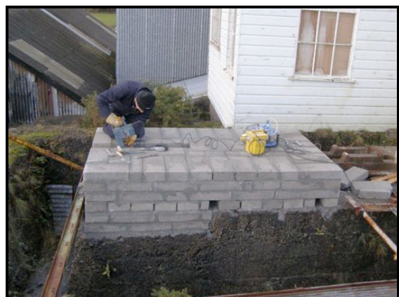
Compressor loadings almost complete December 2009
