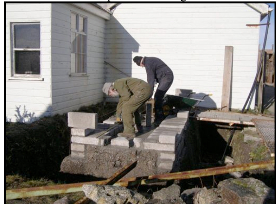
David Blight and Frank Kneebone at work on the compressor loadings
